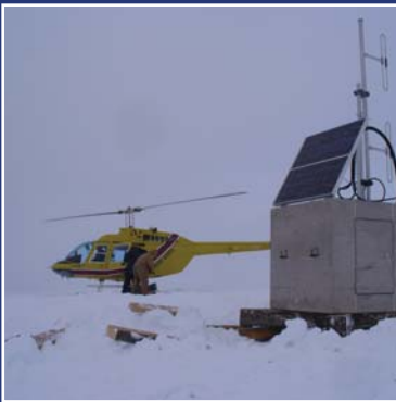
Top: Joe Muff Installs a Strata dish at Quartz Lake
